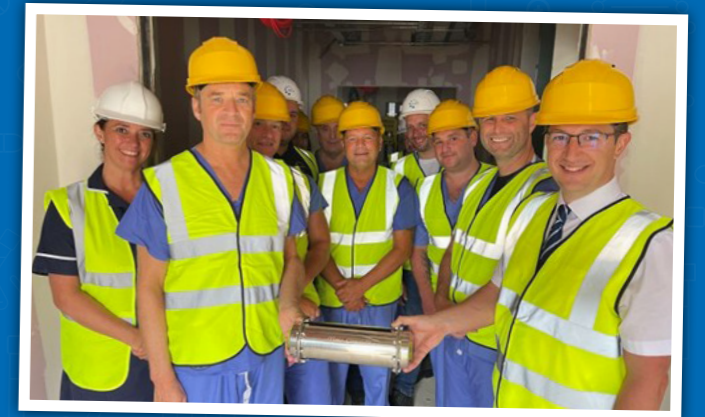
Workers on the building of the Cheshire and Merseyside Surgical Centre phase 2 embedded a time capsule with their chosen mementoes from the present day, into the structure, to commemorate its completion.
